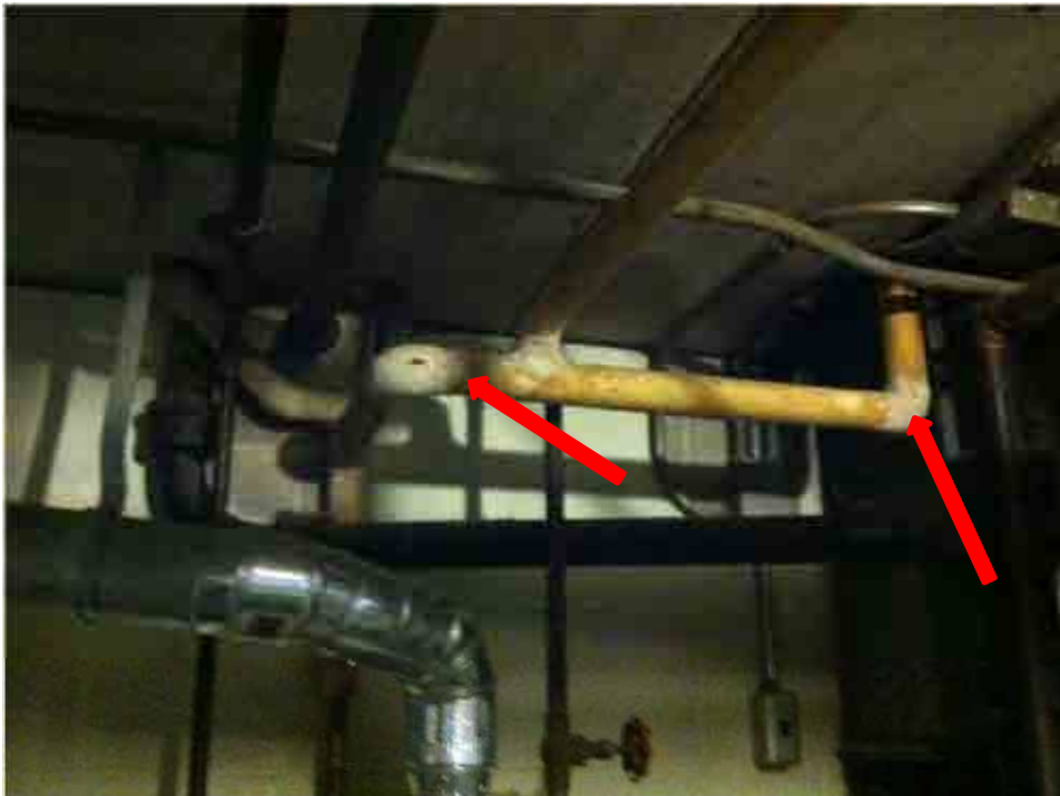
Photo 2 – ACM Pipe Fitting Insulation
